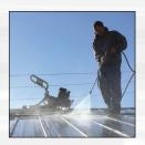
**STEP 1:** Clean the roof surface with **115 Cleaner** and lightly pressure wash.
