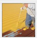
**STEP 2:** Apply **A-125 Metal Roof Primer** to entire substrate prior to coating.
