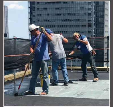
Application with 3/8" nap roller
