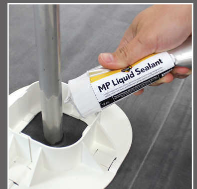
Applying to a pitch pan.
