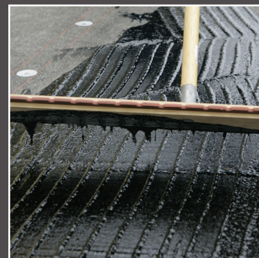
Mule-Hide #102 Fibrated Roof Coating being applied with a squeegee.
