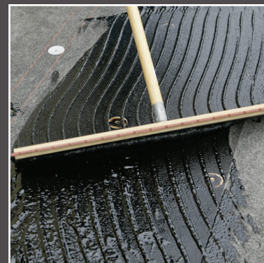
Mule-Hide #111 Non-Fibrated Roof Coating being applied with a squeegee.
