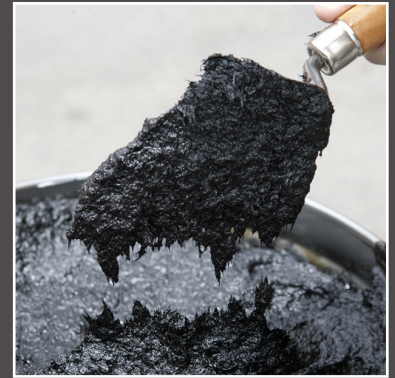
Mule-Hide #211 Plastic Cement being applied with a trowel.
