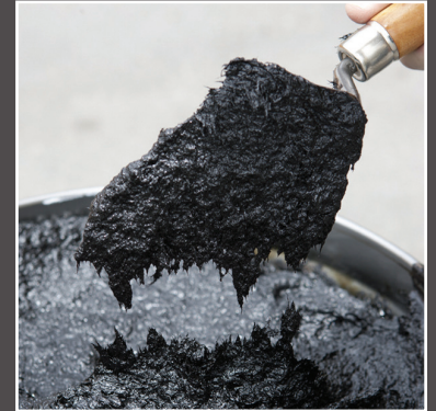
Mule-Hide #221 Wet/Dry Roof Cement being applied with a trowel.
