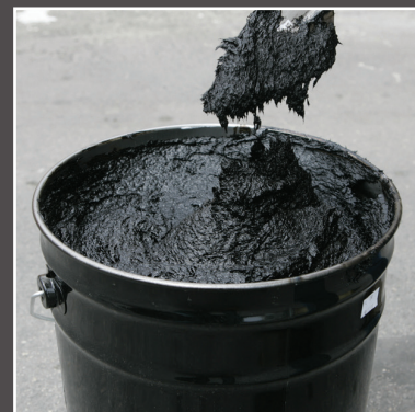
Mule-Hide #231 Flashing Cement being applied with a trowel.
