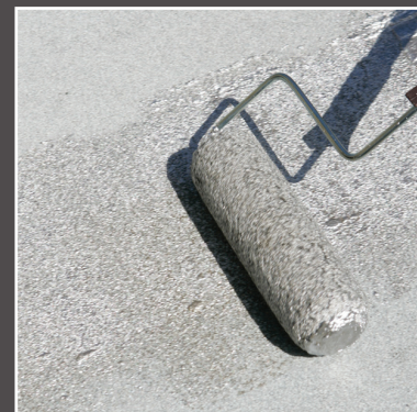
Mule-Hide #406 Standard Fibrated Aluminum Roof Coating being applied with a roller.
