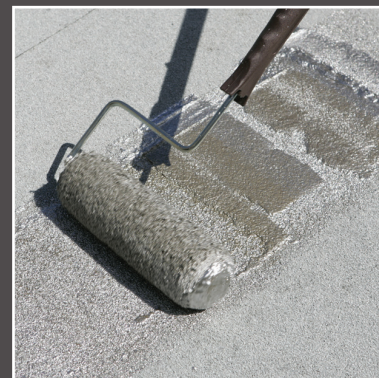
Mule-Hide #410 Premium Non-Fibrated Aluminum Roof Coating being applied with a roller.
