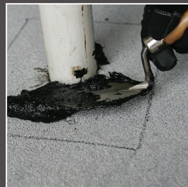
Mule-Hide #421 Mod Bit Adhesive – Trowel Grade being applied with a trowel.
