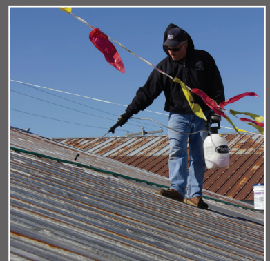
Using airless sprayer.
