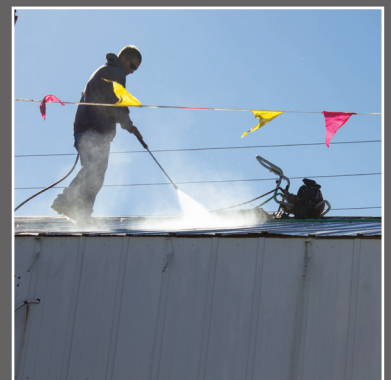
Power washing metal roof.
