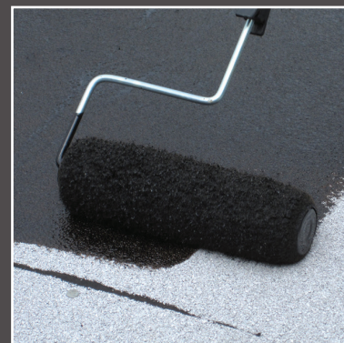
Mule-Hide #121 Asphalt Primer being applied with a roller.
