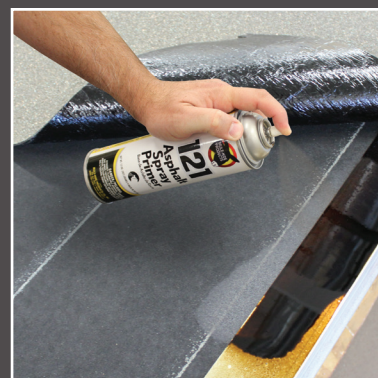
Mule-Hide #121 Asphalt Primer being applied with a spray can.
