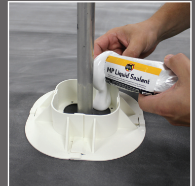
Horizontal installation with MP Liquid Sealant
