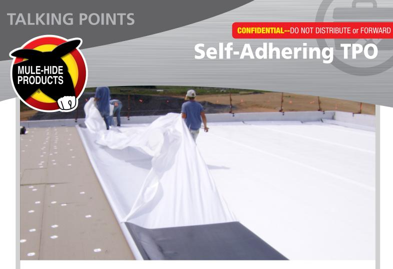
SA-TPO is a 60 mil white TPO membrane laminated to a pressure-sensitive adhesive. It is packaged in  $10' \times 50'$  or  $10' \times 100'$  rolls. There is no lead time on this product, and it can be top loaded with other TPO or EPDM orders shipped from Carlisle, Penn., Senatobia, Miss., and Tooele, Utah.
